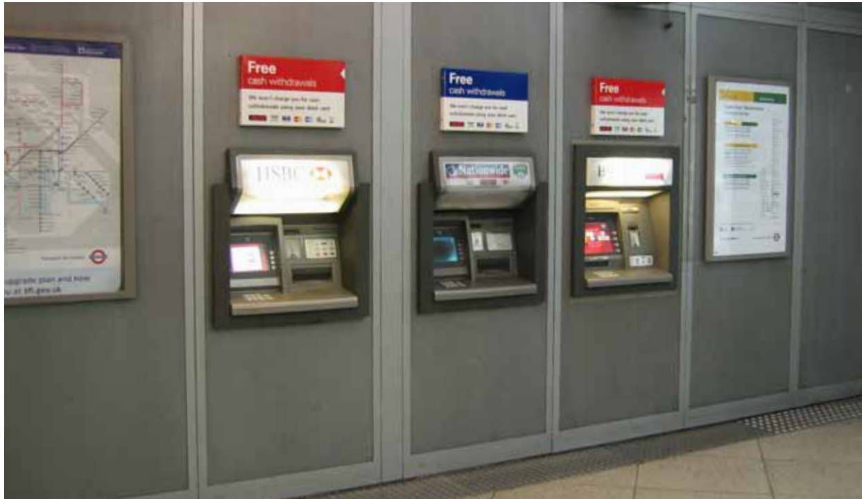
Typical ATM site
